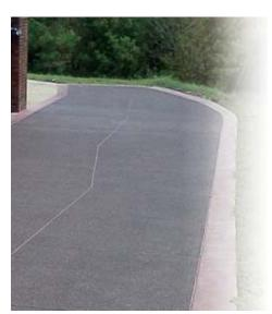
Exposee is a spray-applied, concrete surface retarder used to produce horizontal decorative exposed aggregate finishes. Applied to fresh concrete, Exposee retards the setting of surface mortar, eliminating the need for sand blasting or acid washing.
