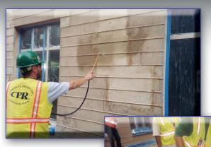
After patching, the walls are treated with a corrosion inhibitor. Then the ChemMasters system is applied.
