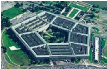
ColorSil with Aquanil Plus 100 water repellent pre-treatment was used on a ten year project to rebuild the Pentagon.
