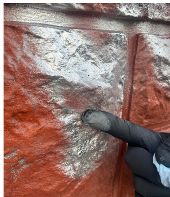
Creates a non-porous surface that resists graffiti adhesion
