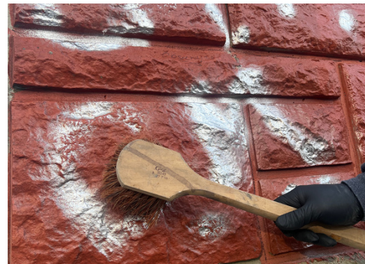
Remove with soap and water with light abrasion
