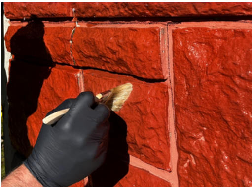
Apply by brush, roll methods, or spray
