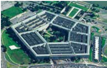
ColorSil with Aquanil Plus 100 water repellent pre-treatment was used on a ten year project to rebuild the Pentagon.
