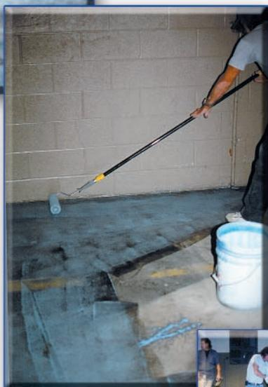
**ChemFlow HS** is a cementitious, self-leveling industrial floor resurfacer designed for interior structural floors. It is a single component, high strength, traffic grade product.
