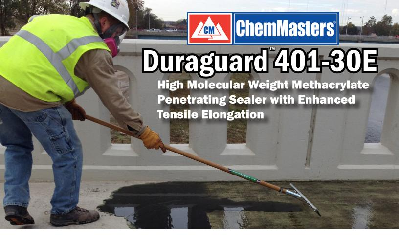
Duraguard 401-30E is a 3-component, low viscosity, solvent free, high molecular weight methacrylate penetrating sealer and crack healer with enhanced tensile elongation for use in high flexural environments.
