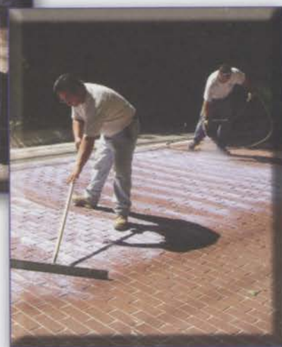
These photos show the various stages of applying ChemMasters Sure-Lock WB over Falls Road.
