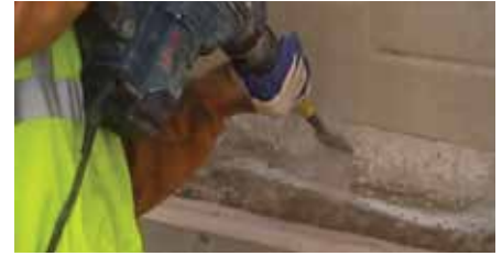
Proper surface preparation is essential to long lasting repairs.
